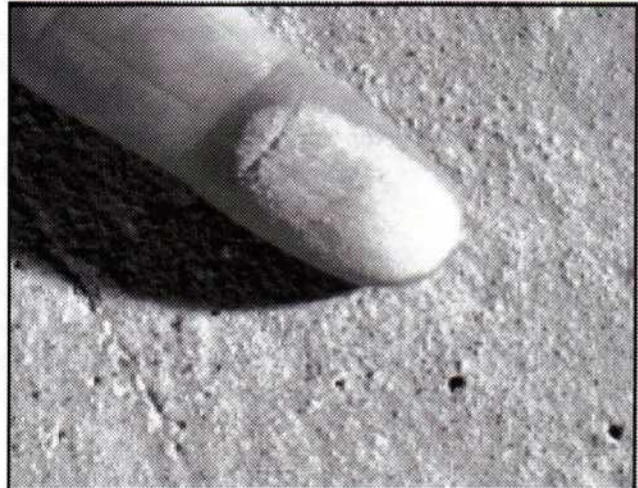
Dusting concrete surface
